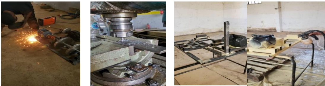
Photos 21, 22, 23: respectively final elements assembly, bolts-way on the reducer support and Applying mastic and painting
